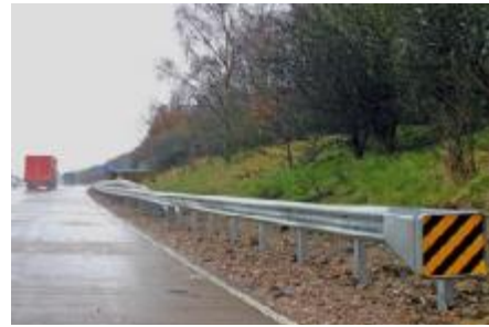
Permanent Safety Barrier
