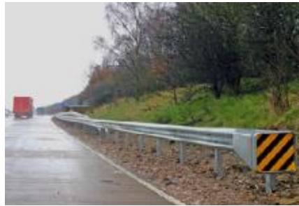
Permanent Safety Barrier
