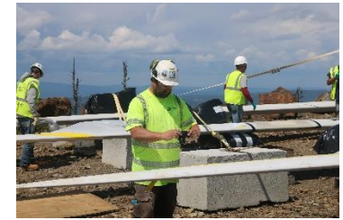
Wind Blade Repair
