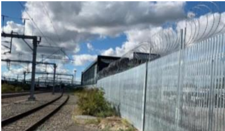
StronGuard™ National Rail Operating Centre
