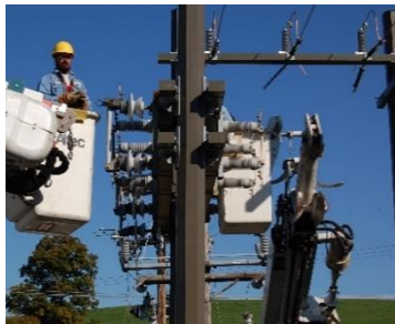
Utility Poles & Crossarms
